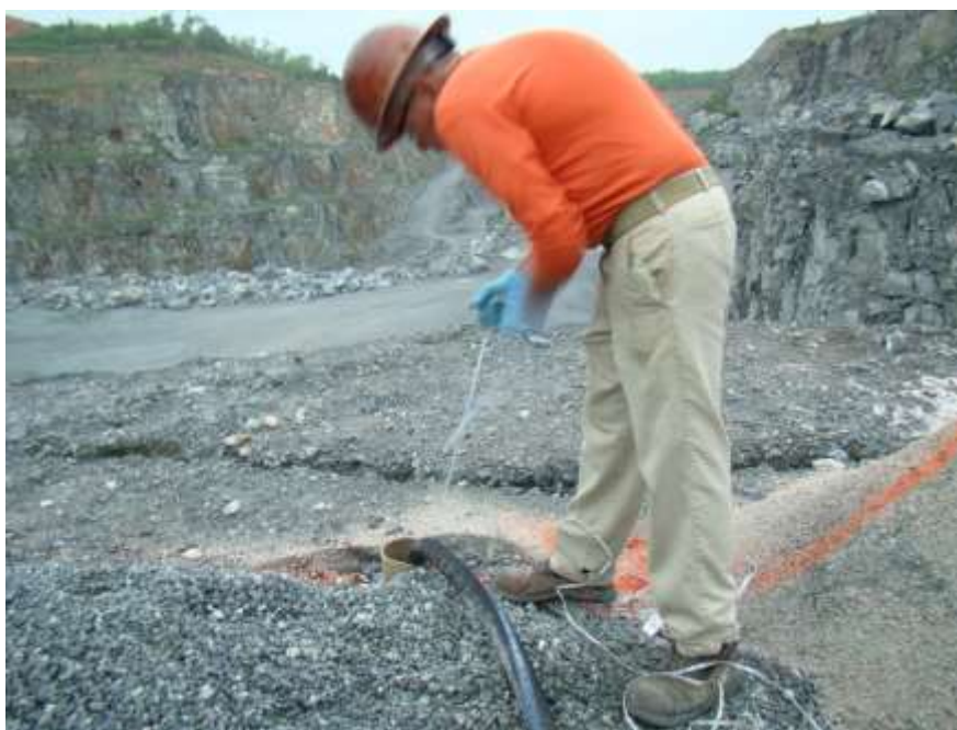
Figure 3.3. Loading a Hole for Test Blast 1 with Titan 1000 SME
