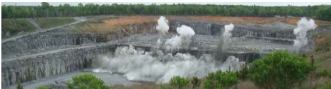
Figure E. 1: April 16, 2015, Shot 1 Blast Photographs
