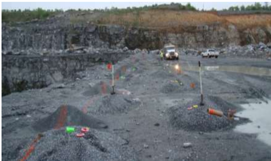
Figure 3.2. Hole Loading During Test Shot 1, with Titan 1000 SME Truck in Background
