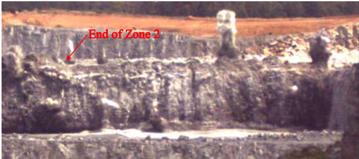
Figure 4.17. Test Blast 4 Movement
